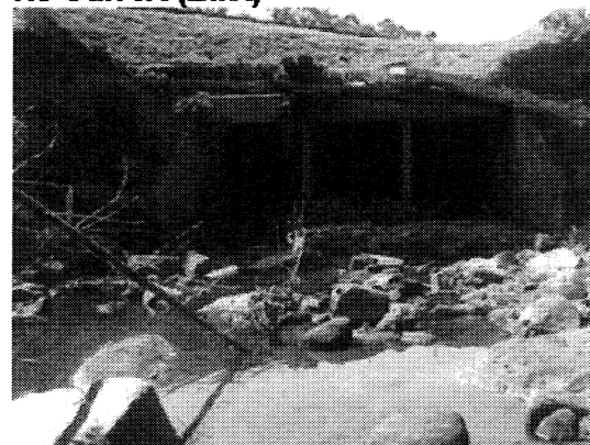
N3 Culvert (East)
