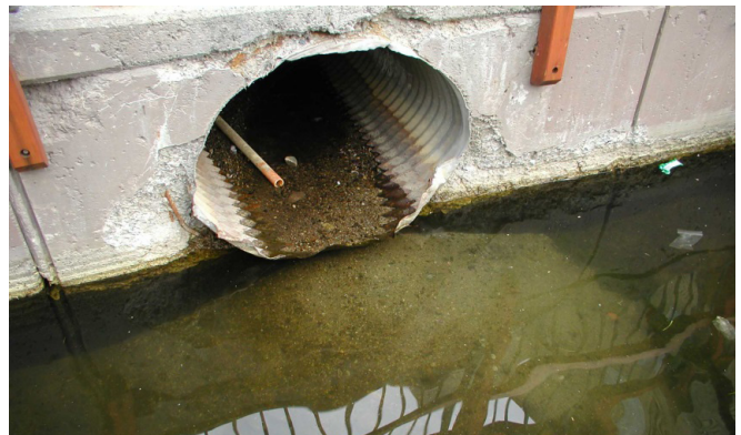
Figure 3 Large particles as bedload and accumulating near outfall in receiving water pond.
