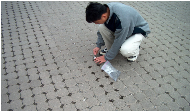
Figure 3 Manual removal and capture of filter and filtrate material in the drainage cells of permeable pavers.
