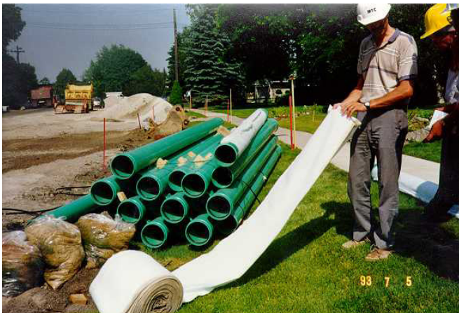
Figure 4 Exfiltration pipes wrapped with nonwoven filter pipe socks.
