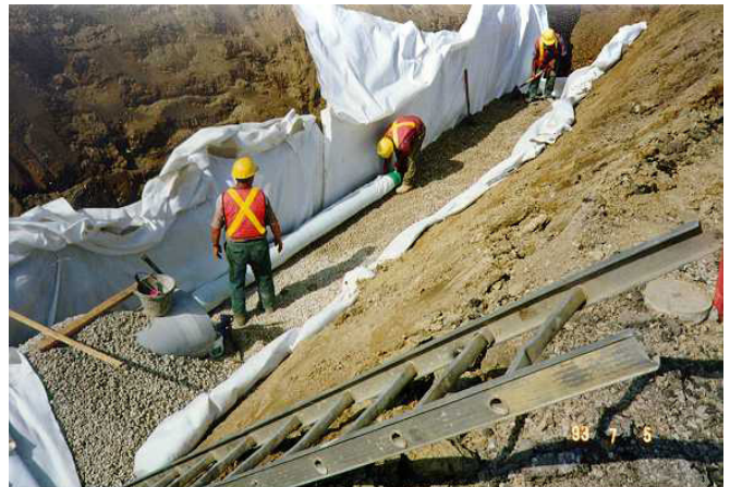
Figure 5 Laying the exfiltration pipes.
