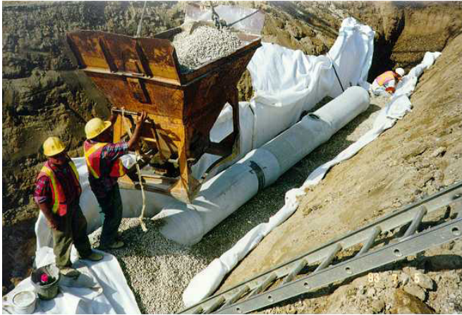
Figure 8 Backfilling the storm sewers.
