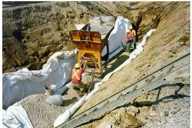
Figure 6 Backfilling the perforated pipes.
