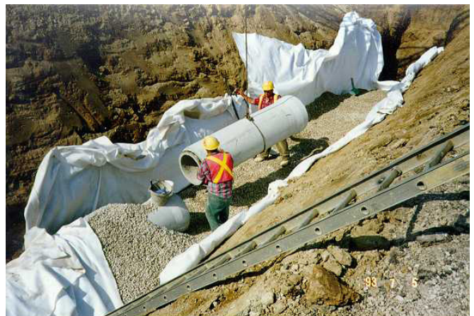
Figure 7 Laying the concrete storm sewers.
