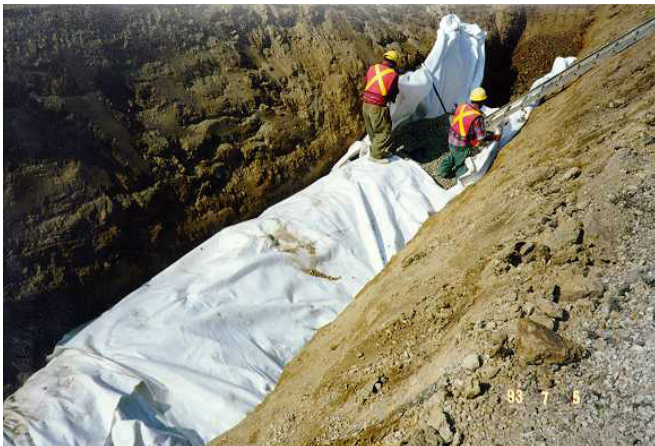
Figure 9 Wrapping the granular trench with nonwoven filter cloths.
